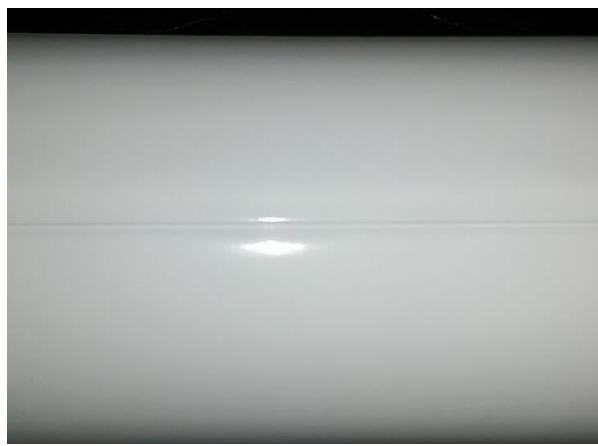
Fig. 2- Mechanical lock forming longitudinal seam
